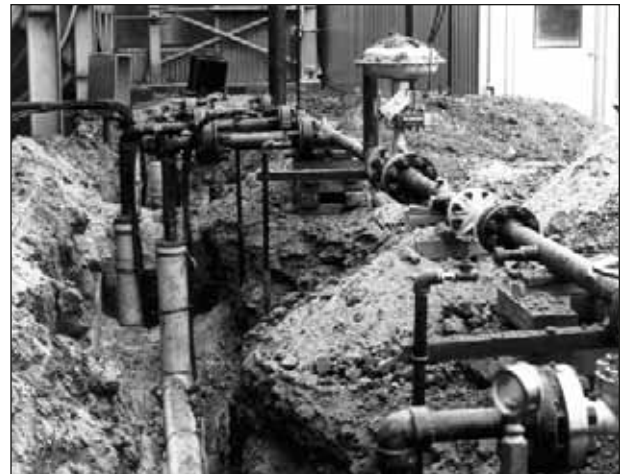
Impedance heating used to heat high temperature, high pressure air for aerospace application.
